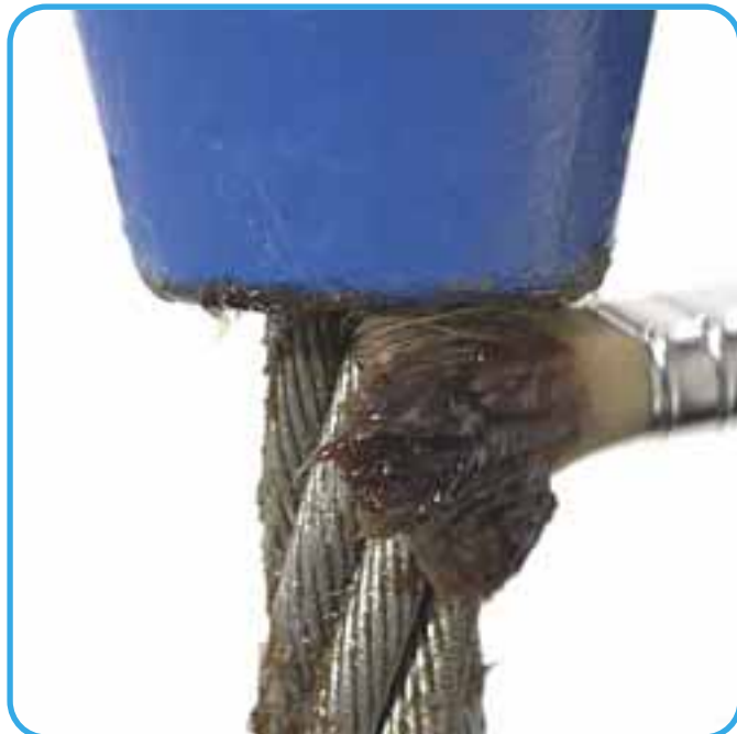
Figure 10: Relubrication of the rope below the socket after removing from the vice.
