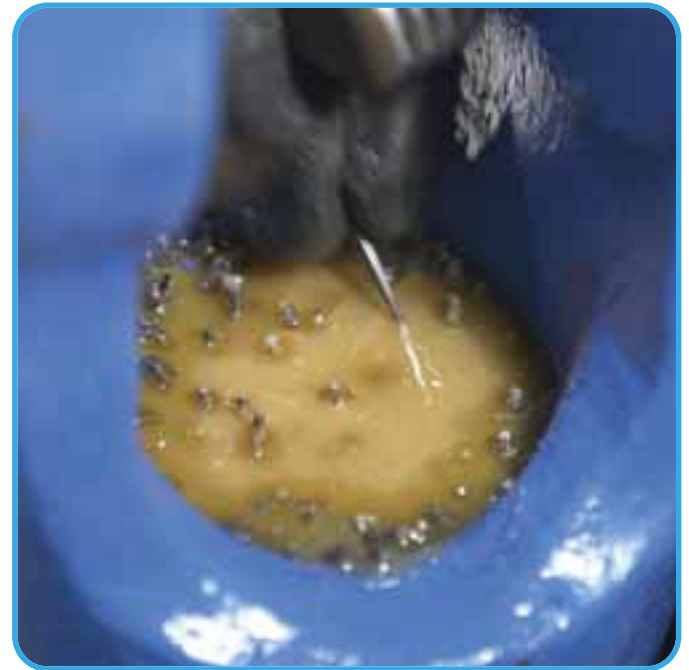
Figure 11: Scratch testing the material in the socket one hour after it has gelled.
